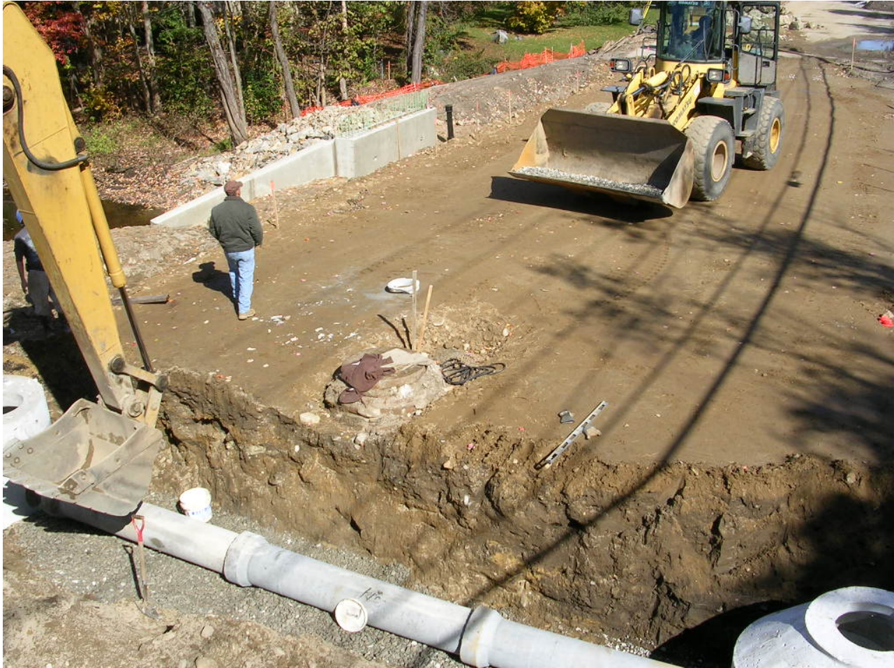
Installing storm drainage
