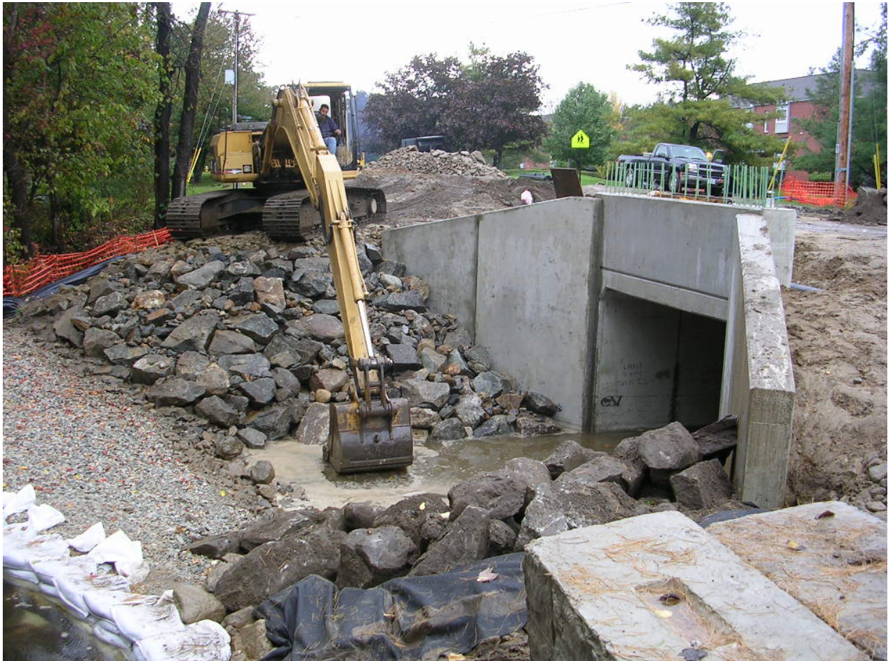
Placing rip rap stone adjacent to bridge
