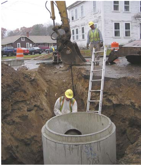
Installation of catch basin and pipe at intersection (above and left)
