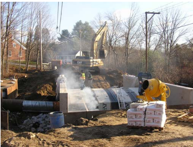
Placement of waterproof membrane on new precast bridge joints (above)
