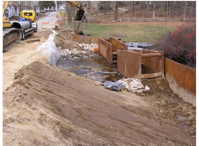
Side slope prep prior to stone placement
