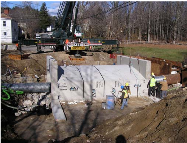
Installation of Precast Concrete Bridge Sections (above)
