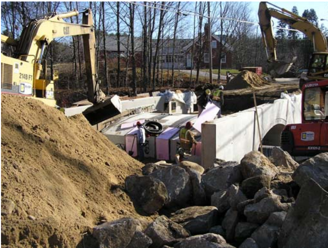
Backfilling against new precast bridge
