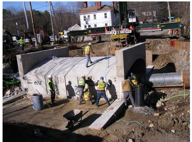
Installation of Precast Concrete Bridge Sections (above)
