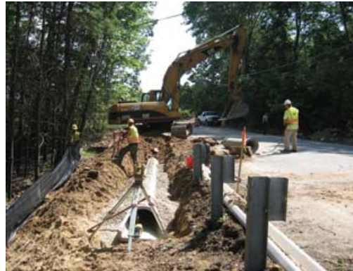
Laser used to install pipe per design specs
