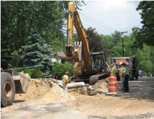
Concrete pipe moved into position by backhoe
