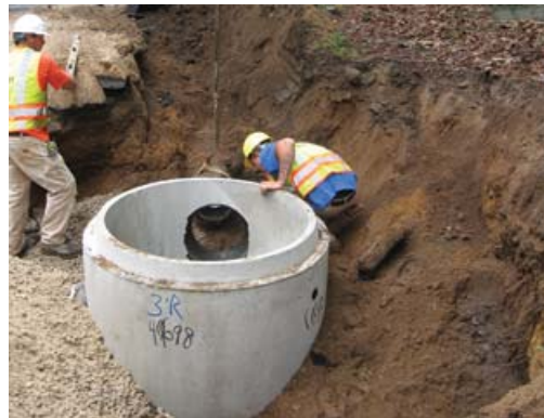
Crew connects drainpipe to new catch basin
