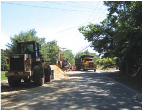
Truck delivers crushed stone to pipe laying crew
