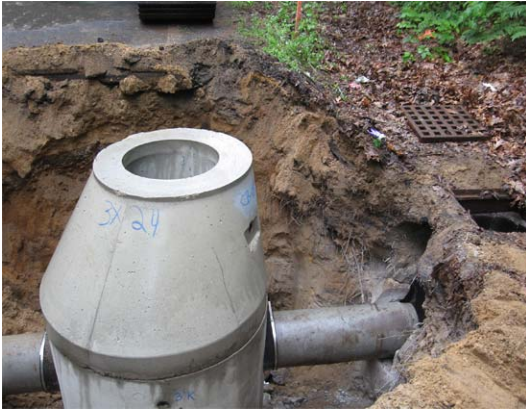
Construction of Catch Basin 18, (near Higgins Lane)
