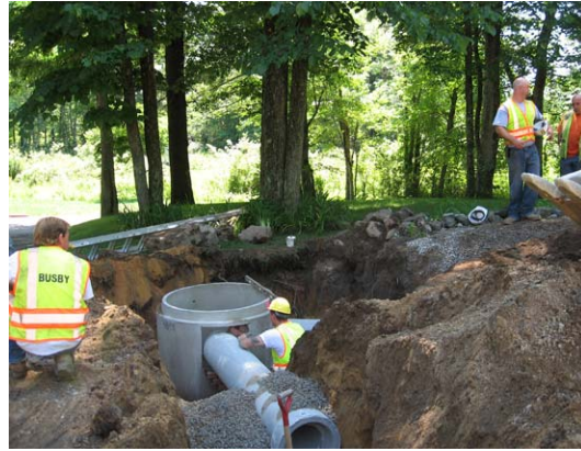
Constructing Catch Basin 20, (near 210 South Main St.)
