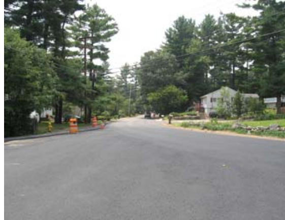
Base coat of pavement in place
