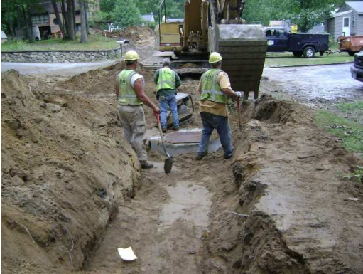
6/05/08 – Drainage Pipe Installation
