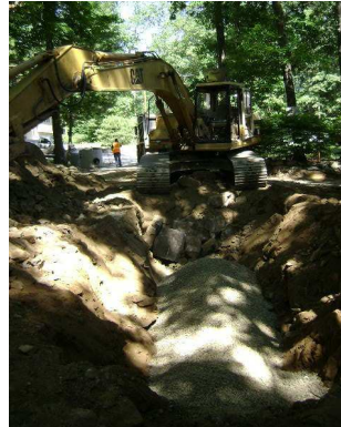
6/13/08 – Drainage Pipe Installation
