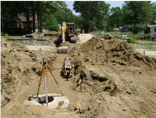
6/10/08 – Catch Basin Installation
