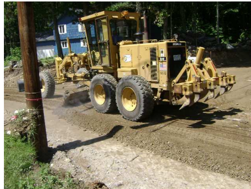
6/25/08 – Crushed Gravel Installation
