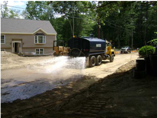
6/19/08 – Dust Control Operations
