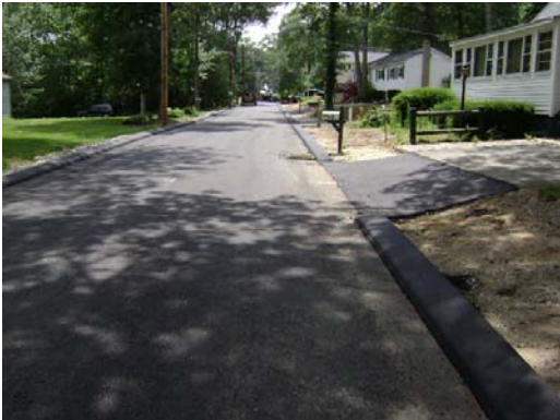
7/17/08 – Berm and Driveway Work
