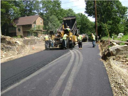
7/02/08 – Binder Course Paving
