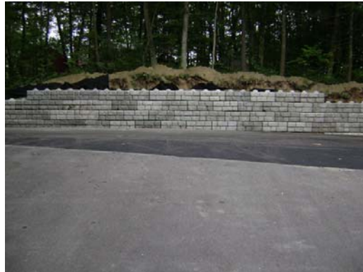
7/22/08 – Retaining Wall Construction
