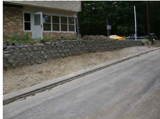
8/04/08 – Retaining Wall Construction
