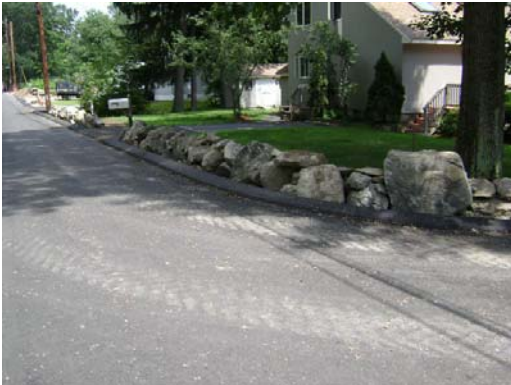
8/01/08 – Stone Wall Reconstruction
