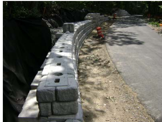
8/01/08 – Retaining Wall Construction
