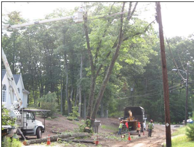
Tree clearing for improved sight distance
