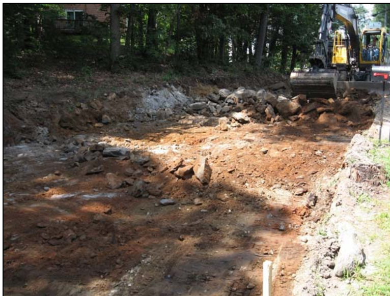
Removal of exiting roadway and sub-base along Shore Drive
