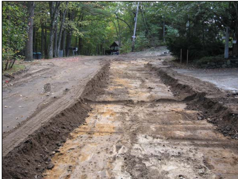
Placement of sub-base material along Shore Drive
