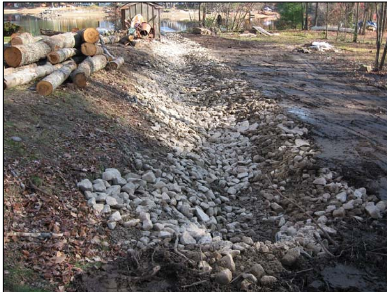
Stone swale conveying drainage to Arlington Pond
