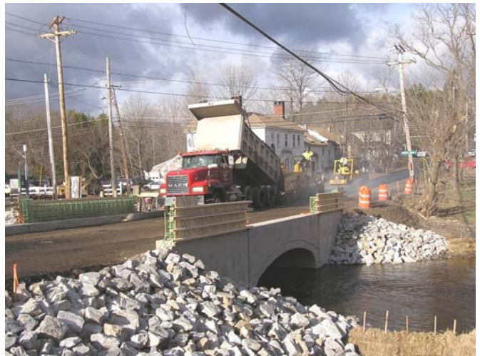
binder course paving of road
