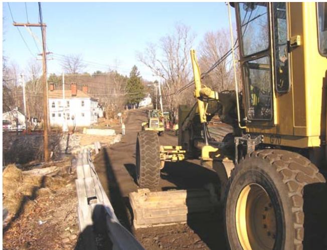
grading and compacting road gravels
