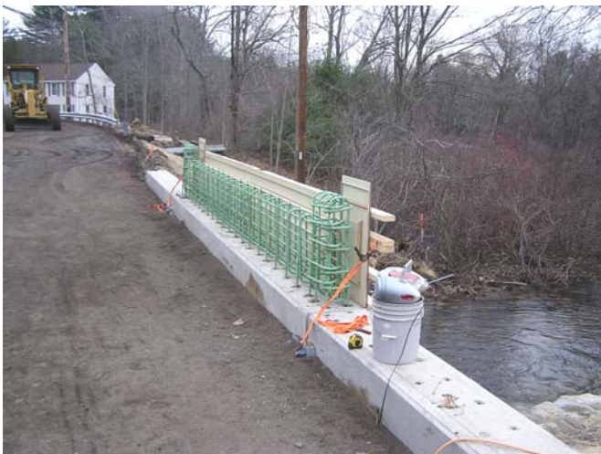
bridge rail reinforcing steel
